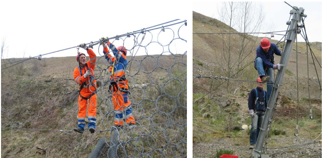
Figure 40 Tension belts between the posts for installing RUNTOP ropes and nets
