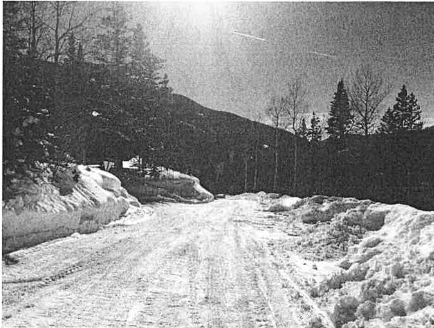
Viewing south on Bull of the Woods Road. Subject Tracts 1 & 2 are on the right.
