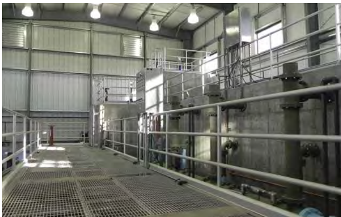
A Blue PRO® installation in Grangeville, Idaho for 0.05 mg/L phosphorus
