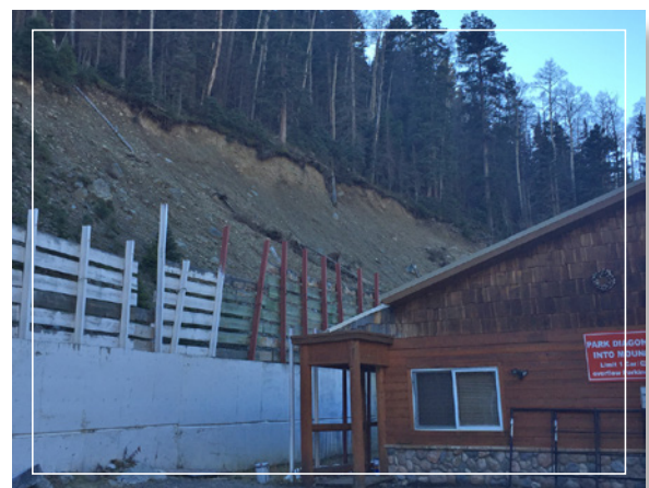
Large cut and fill increases the risks of landslides and erosion
