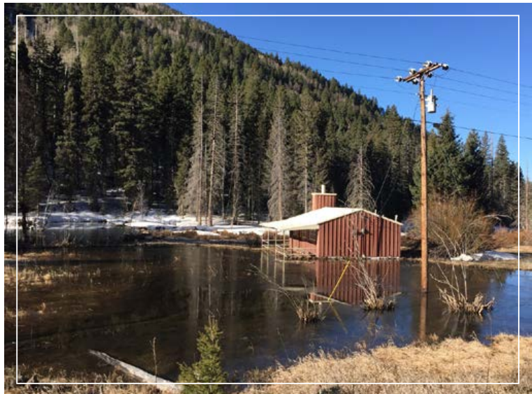
Flooding along Highway 150
