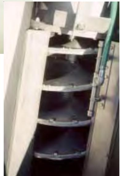
*The stainless steel, shaftless screw conveyor improves screening performance.*
