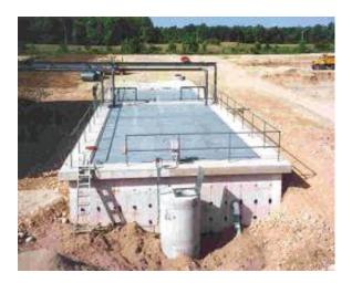
The total power consumption for a 1.0 MGD conventional SBR plus aerobic digestion would be approximately 1,680 KWH/day. The total power consumption for a 1.0 MGD ISAM<sup>TM</sup> SBR is approximately 845 KWH/day; 50% less than a conventional SBR.
