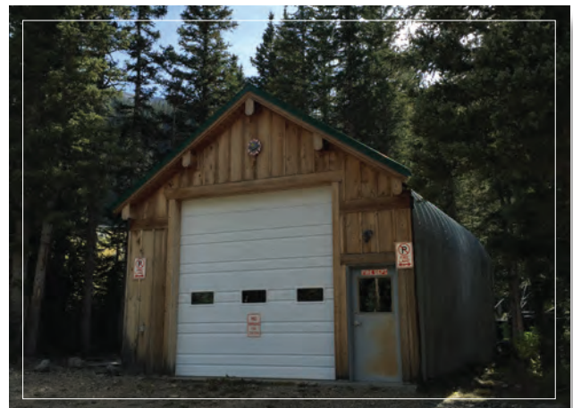
Fire Substation #2. The Village leases the property underneath the substation from TSV, Inc.
