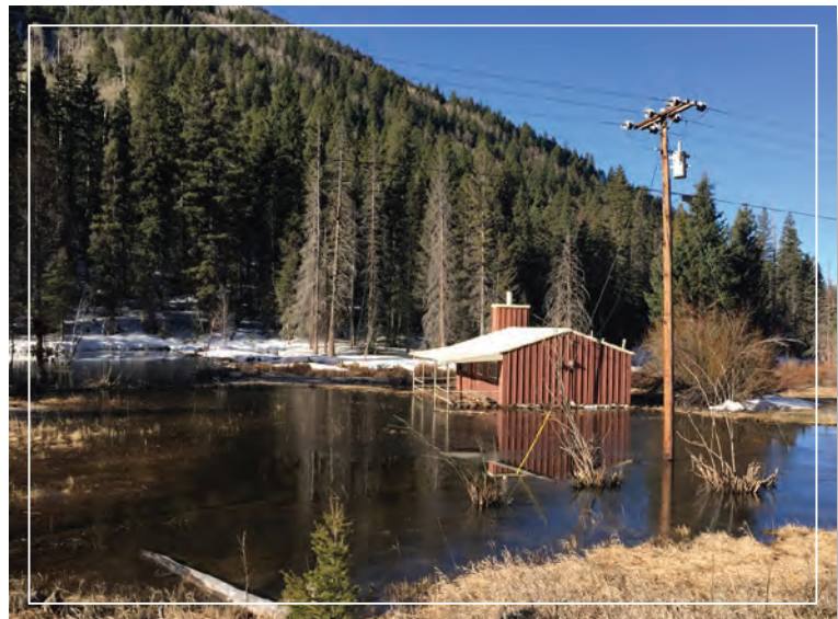
Flooding along Highway 150
