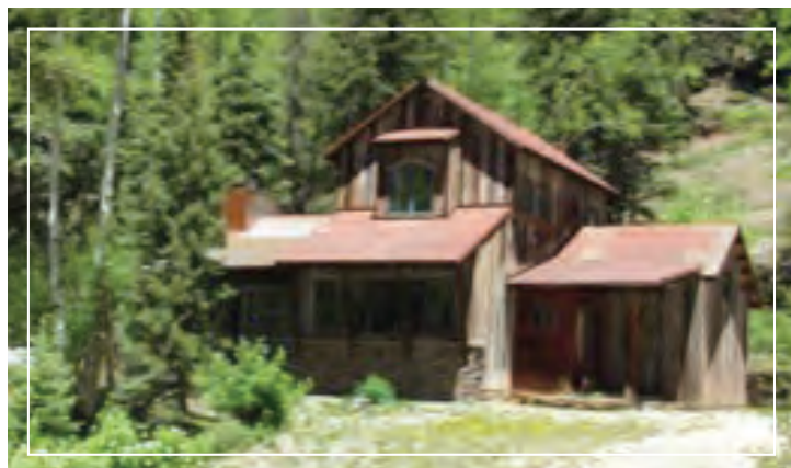
Residence, Cliffhanger Loop Road
