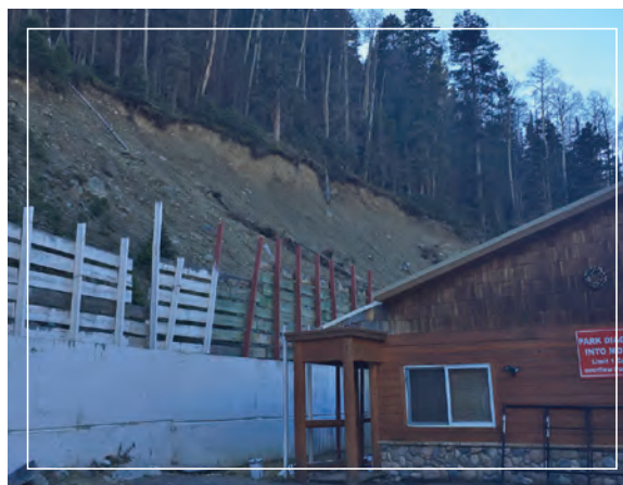
Large cut and fill increases the risks of landslides and erosion
