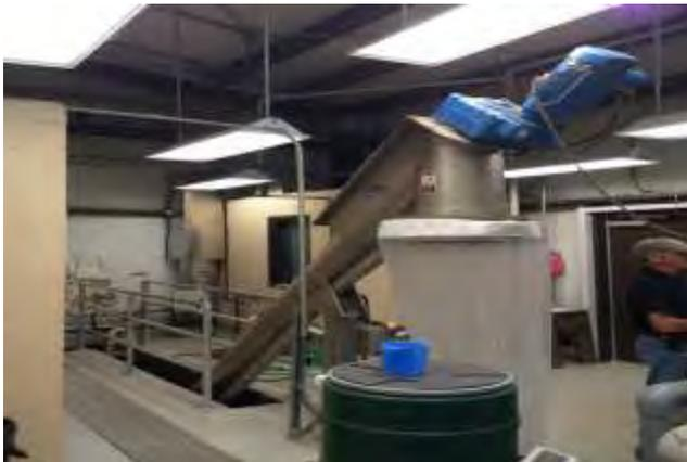
The screen assembly consists of a stainless steel cylindrical fine screen with  $\frac{1}{4}$ -inch bar spacing and a nylon cleaning brush, screw conveyor, and a compaction dewatering cone, and discharge chute. Screenings are swept by the brush assembly into the screw conveyor. Within the conveyor, the screenings are washed, compacted and dewatered, and then dropped into a hopper.
