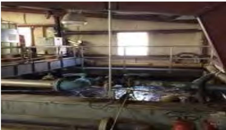
The selector pumps convey nitrate-rich internal recycle flows to Basin 1 to utilize the additional denitrification capacity at a recycle ratio of 5:1 in the summer and 3:1 in the winter (3-5Q recycle: 1Q influent). RAS flows have been typically maintained at a ratio of 0.6 to 0.9 RAS:influent Q. The MLSS in Anoxic Basin 4B is maintained in suspension using a submersible mixer, and MicroC 2000 is dosed, if
