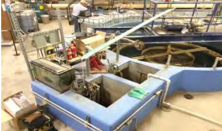
The RAS/WAS pumps are 4-inch submersible pumps sized at approximately 5 Hp, with a design point of 300 gpm at 22 ft. The pumps are equipped with VFDs to allow a turndown of approximately 50 percent. The RAS return rate is typically in the range of 0.6 – 0.9 times the influent rate (0.6 - 0.9Q). It is believed that the current RAS rate is a contributing factor to the observed clarifier bulking issue.
