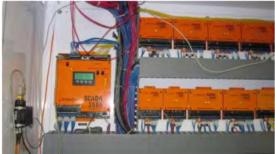
The 2005 improvements project included a Main Control Panel (SCADA-301) which has the majority of the Plant Inputs and Outputs (I/O) run to the main control panel. The plant I/O is terminated on I/O cards which are a component of the Sensaphone SCADA 3000 system. All signals are run in individual wires/conduits; there are no Ethernet communications between areas in the facility.
