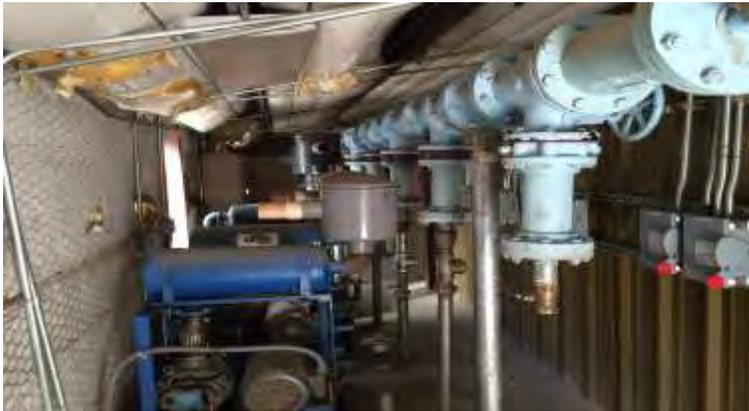
The 6-inch discharge header runs from the blower room to feed a 4-inch Tee to Basin 4A and a 10-inch Tee to the aeration basins. Air to the grid in each basin is controlled by butterfly valves located at the side of each basin. Based on information provided by the District, the installed blower capacities used for the activated sludge process aeration are:
